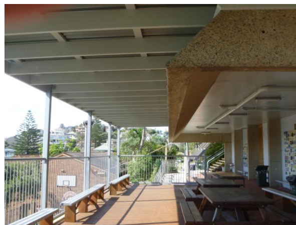
Roof completed to provide shade for lunch area on deck
