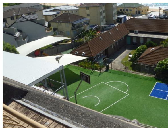
Shade structures and replacement playground surface built during 2010
